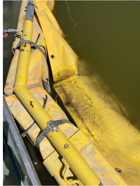
Broken zip ties
